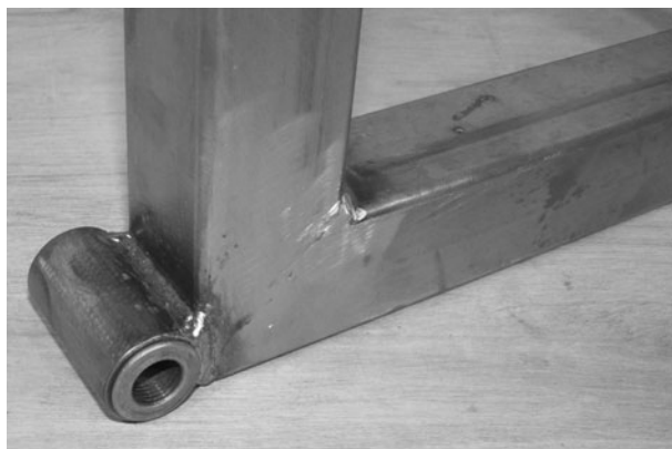
Figure 12-38 Pivot tube welded in place
