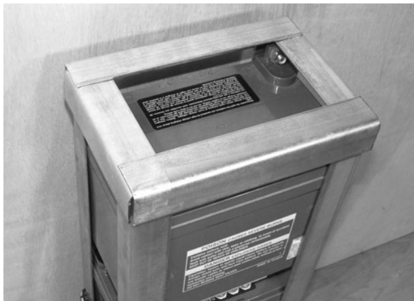
Figure 12-8 Cutting the battery pack base
