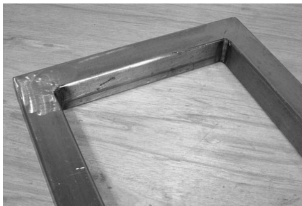
Figure 12-18 Cleaning the center frame welds
