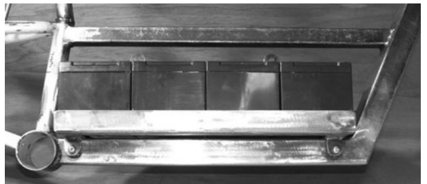
Figure 13-52 Battery tab nuts and bolts in place
