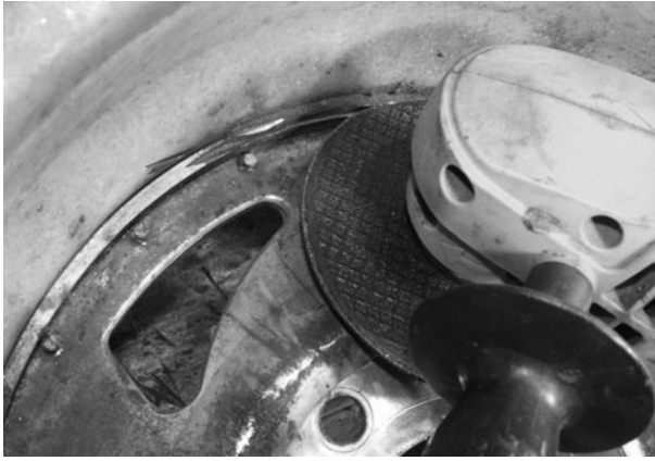
Figure 2-3 Grinding out the welds
