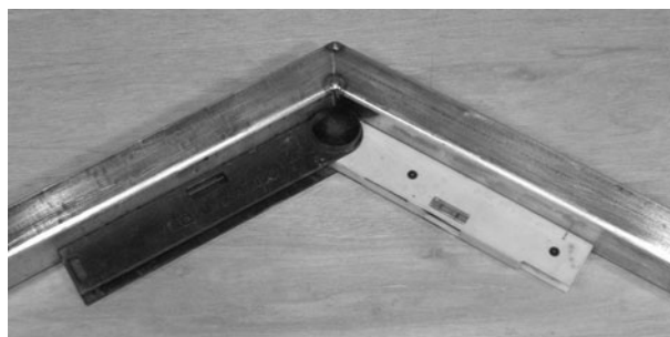
Figure 13-23 Tack welding the boom tubes
