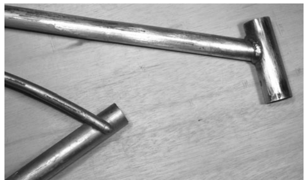
Figure 3-5 Cleaning up the welded area
