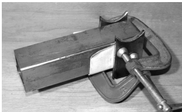
Figure 5-87 Setting up the plates for welding
