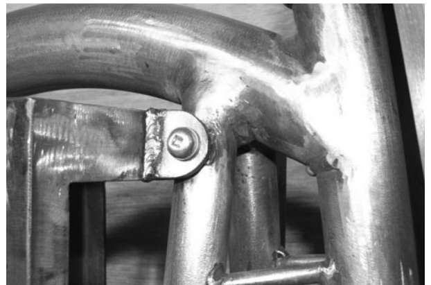
Figure 11-87 Battery box bolted onto the frame
