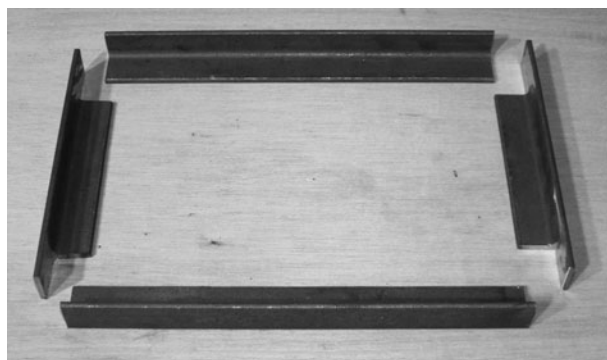
Figure 11-2 The base for the battery box
