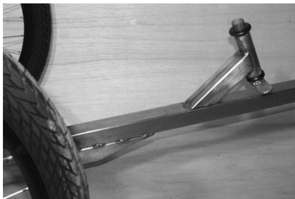
Figure 6-89 Tack welding the steering support tube in place
