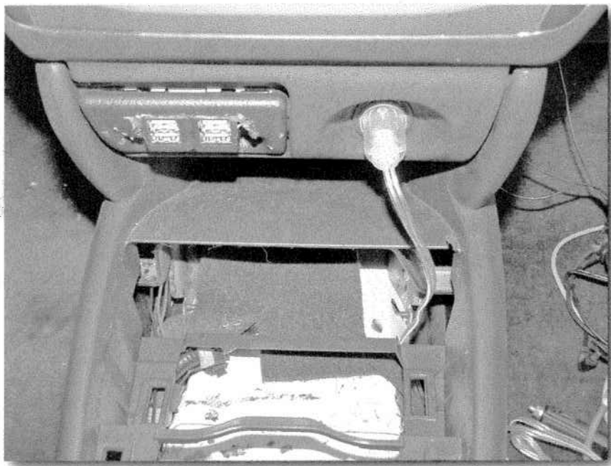
FIGURE 5-11: Running the power cable under the center console.
