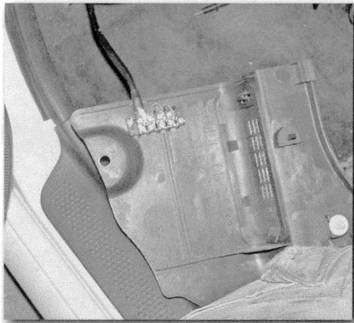
FIGURE 3-27: The barrier terminal strip connected to the fuse box cover.
